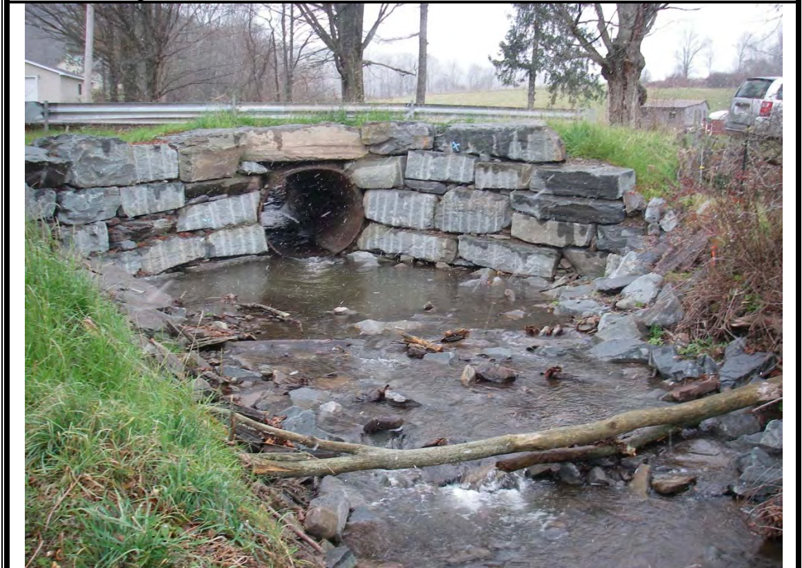
Photo 6: Looking upstream after construction of stacked rock headwalls and plunge pool.
