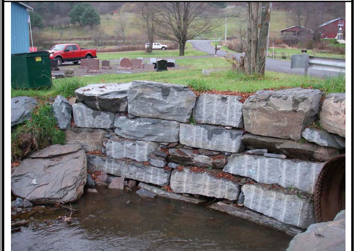
Photo 4: Looking from left streambank at stacked rock headwall.
