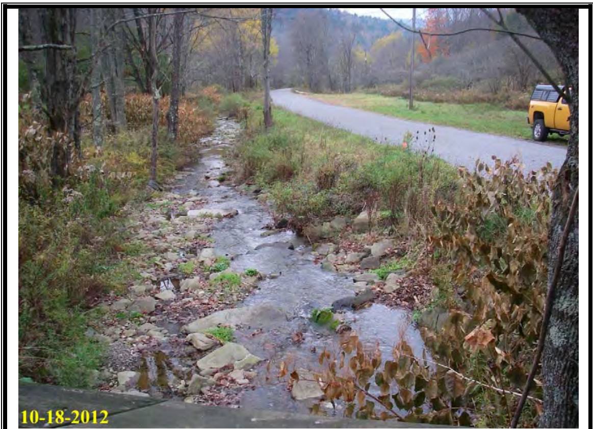
Photo 5: Before construction, looking downstream from private bridge.
