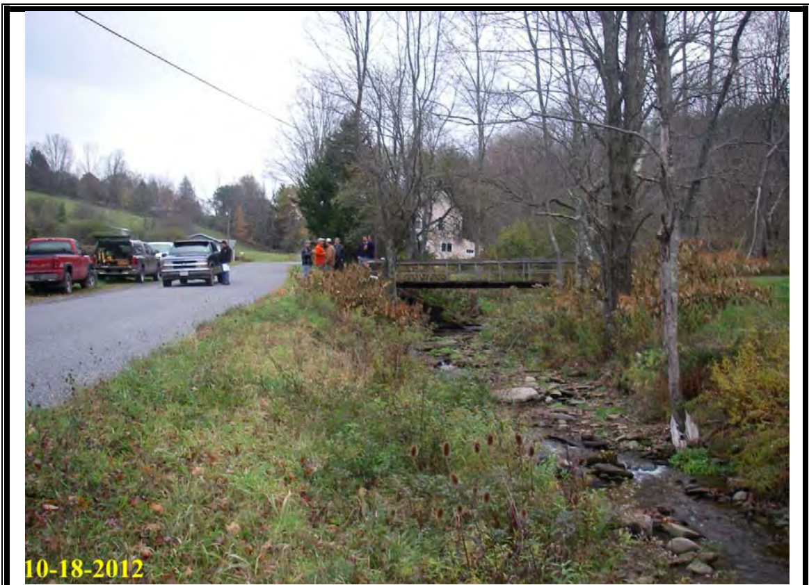
Photo 7: Before construction, looking upstream from right streambank.
