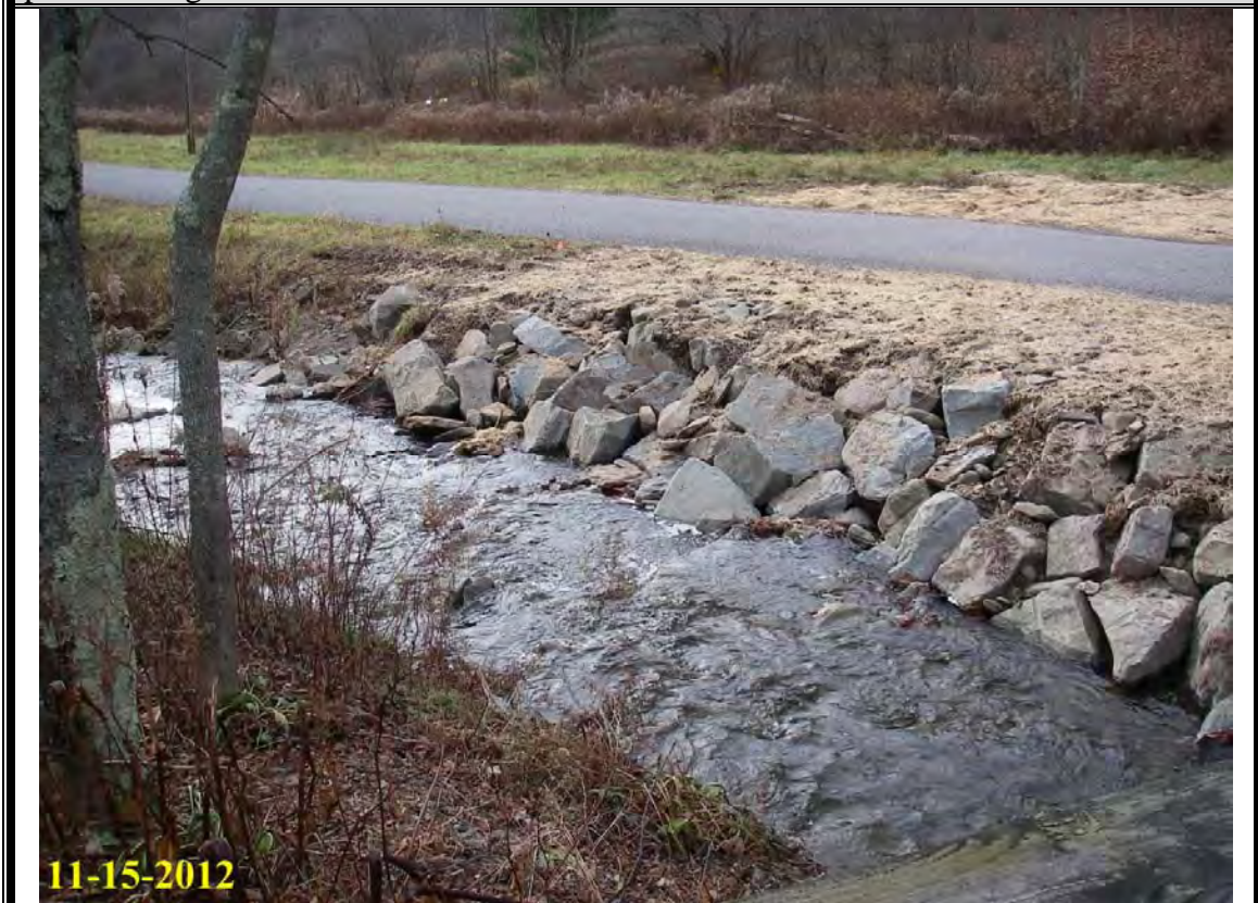
Photo 2: After construction, looking downstream from left streambank standing on private bridge.
