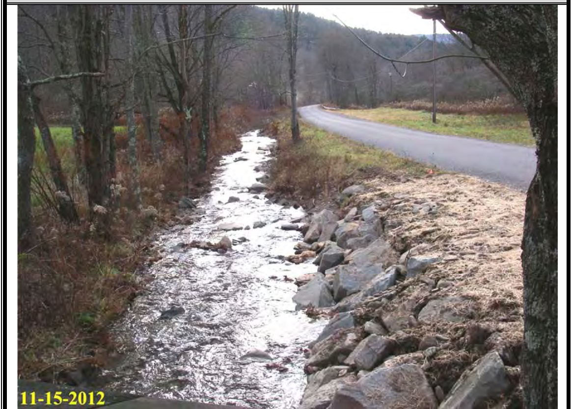
Photo 6: After construction, looking downstream from private bridge.
