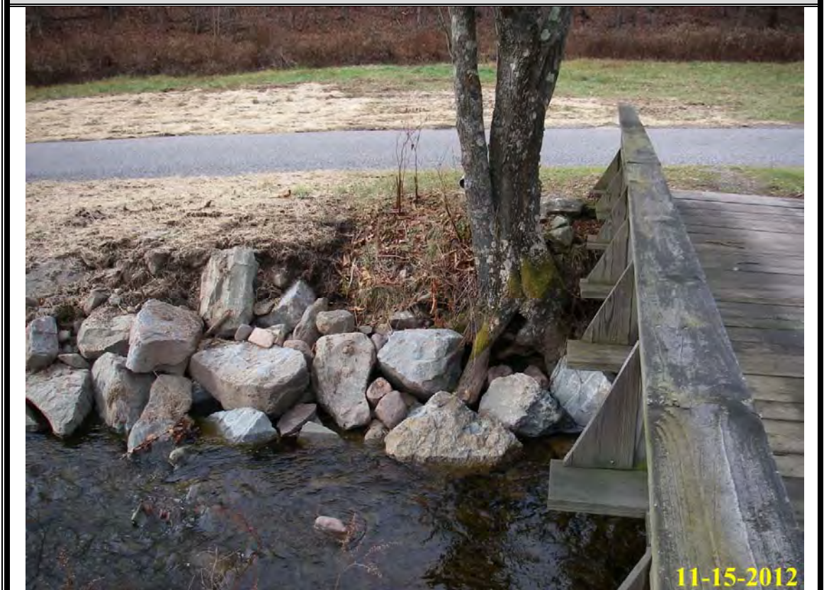
Photo 4: After construction, looking at right streambank standing on private bridge.
