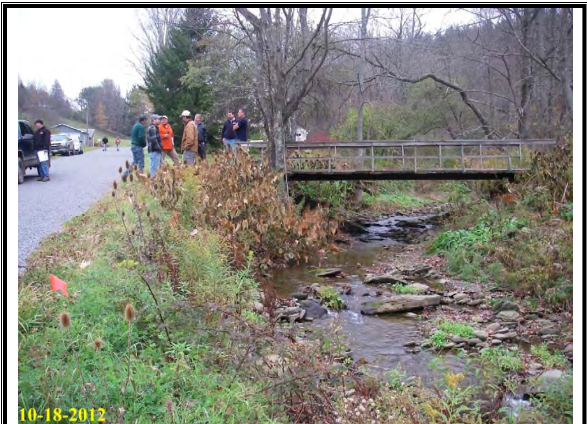
Photo 9: Before construction, looking upstream from right streambank at lower portion of the project.
