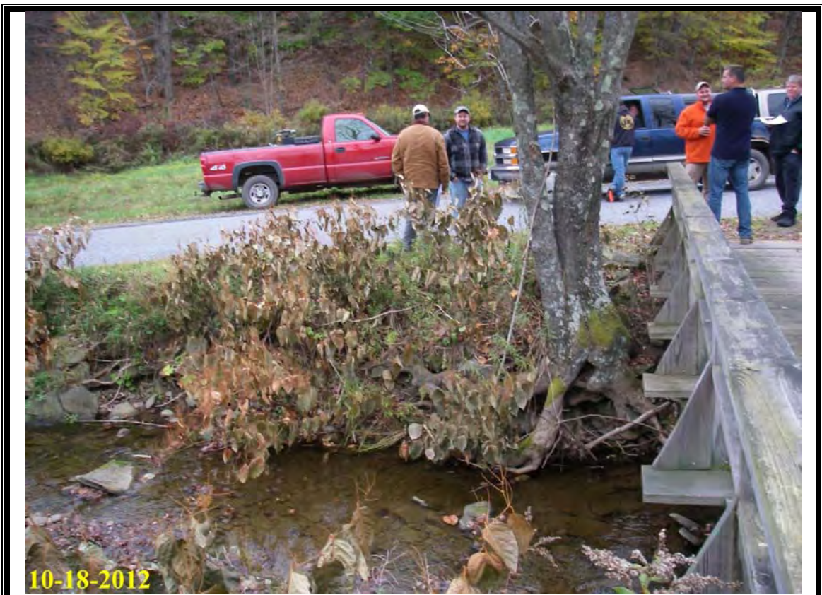
Photo 3: Before construction, looking at right streambank standing on private bridge.
