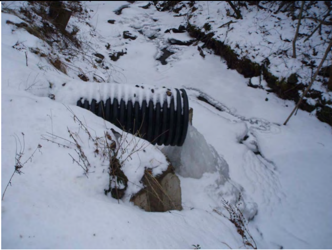
Photo 9: Looking upstream from right streambank at Site C and culvert outlet causing erosion.
