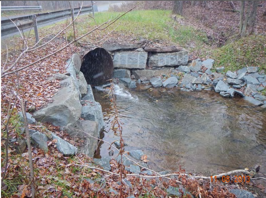
Photo 6: Looking at culvert after construction of stacked stone headwalls.
