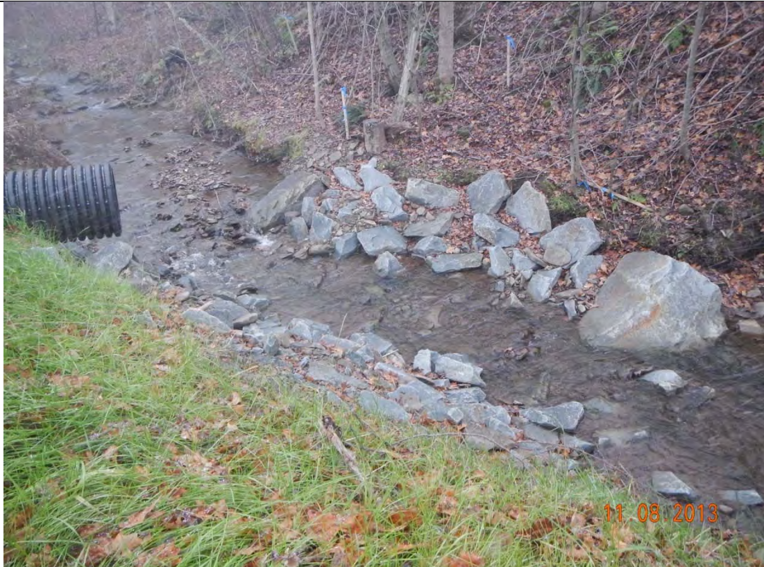
Photo 10: Looking upstream from right streambank after construction of culvert outfall protection and hardened riffle structure.
