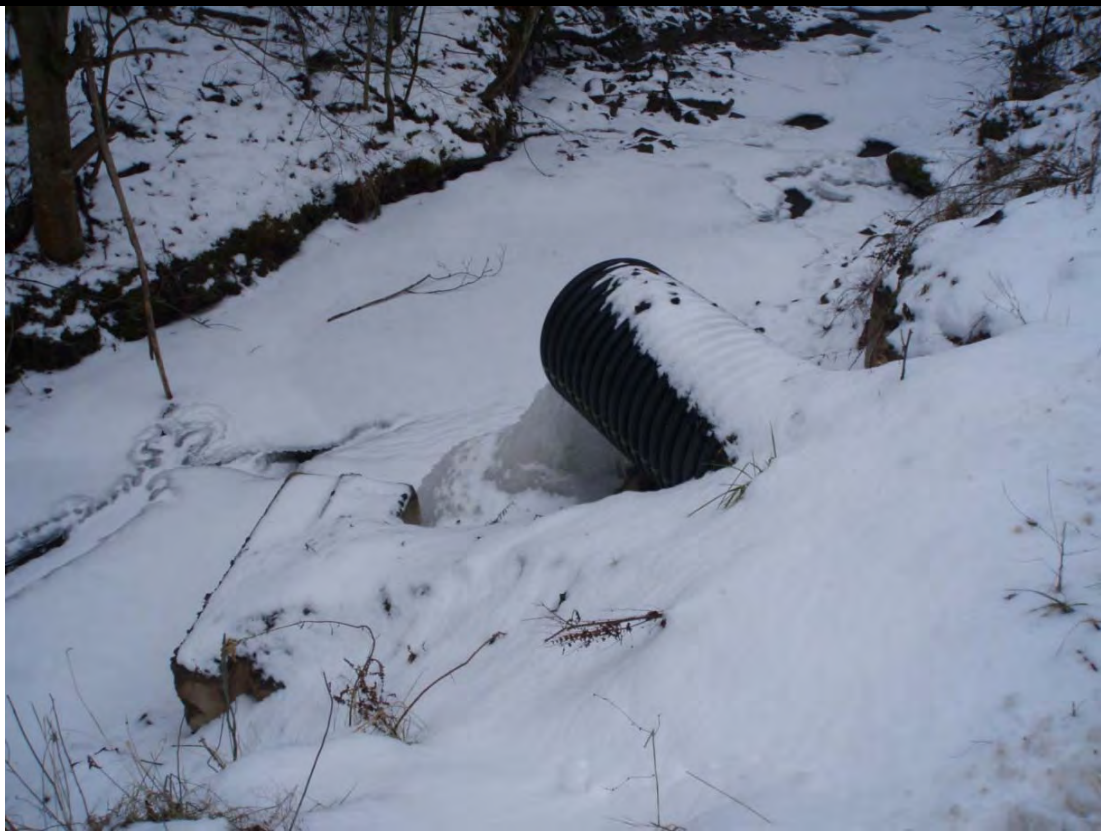
Photo 11: Looking downstream from right streambank at Site C and culvert outlet causing erosion.
