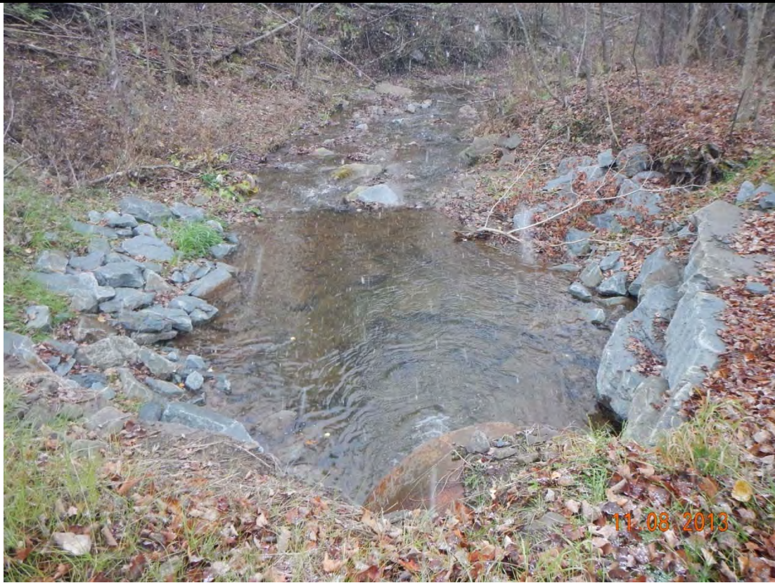
Photo 7: Looking downstream from MacGibbon Hollow culvert after construction of stacked rock headwalls.
