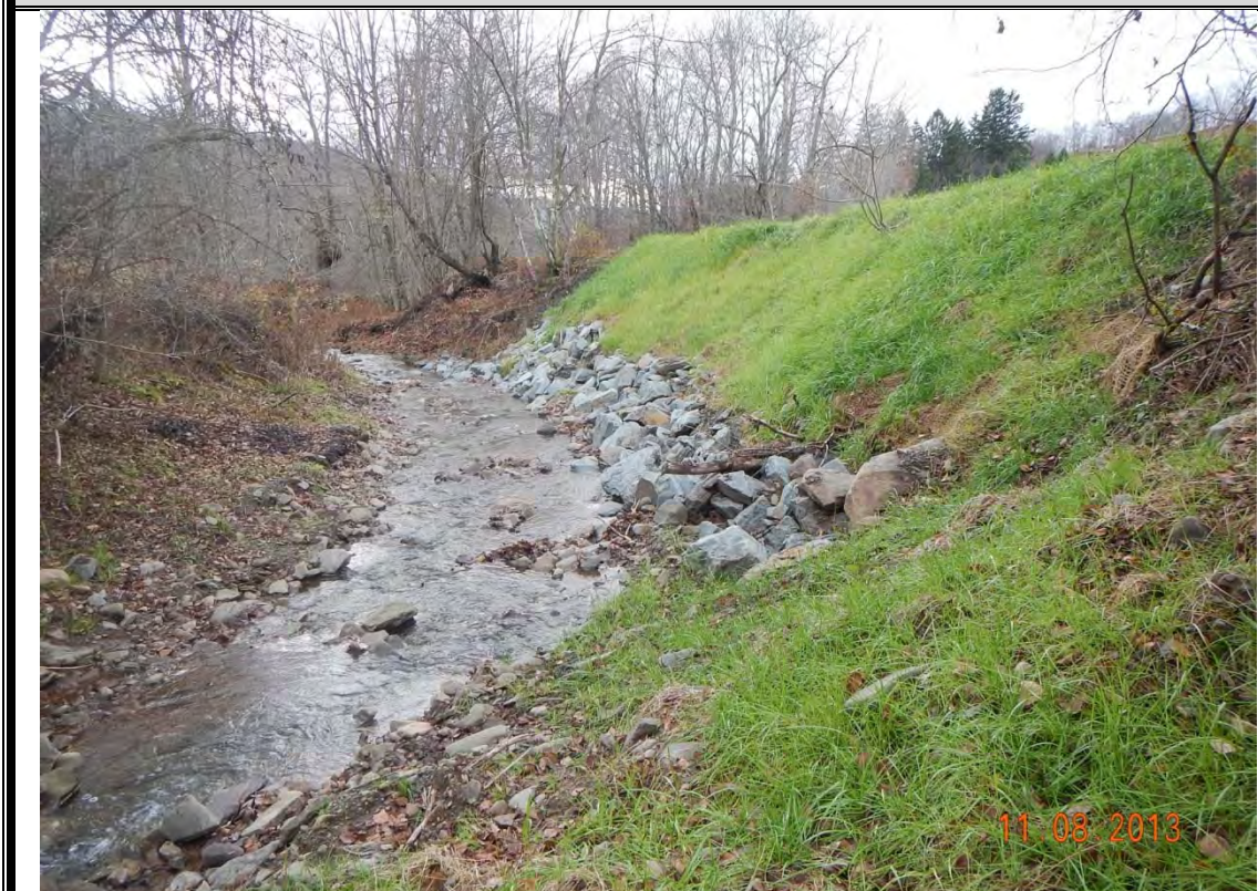
Photo 16: Looking downstream from right streambank after construction of rock rip rap.
