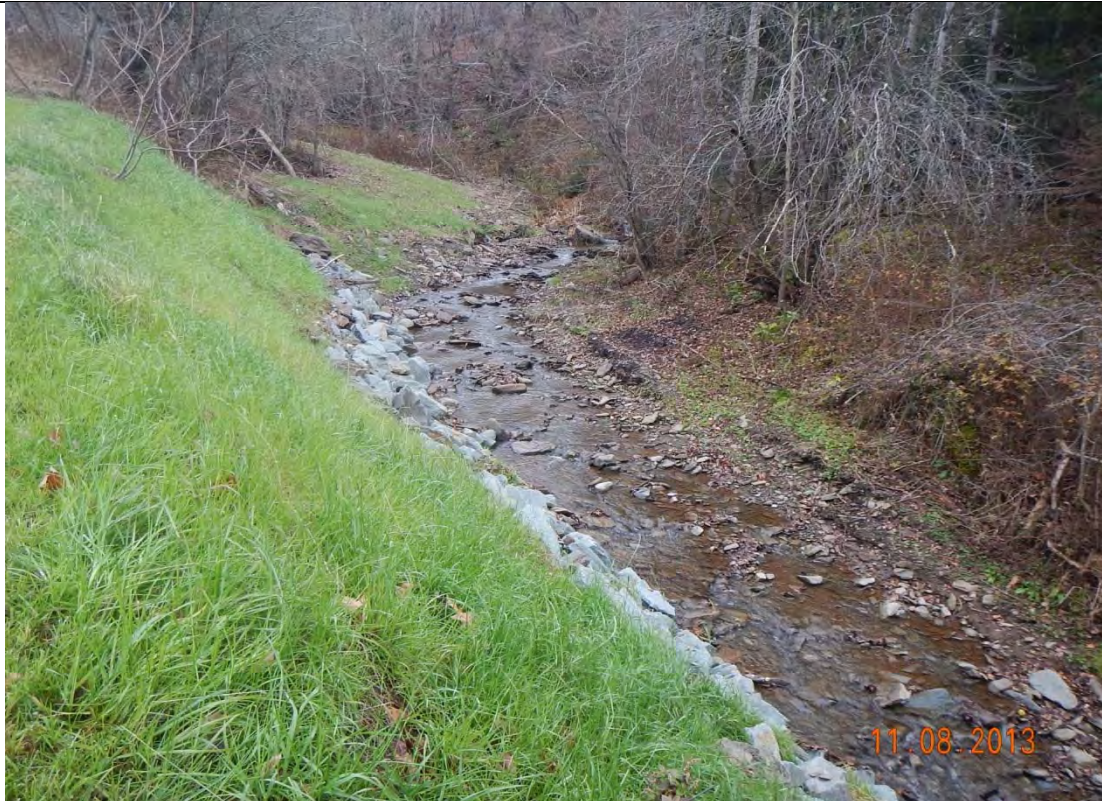
Photo 14: Looking upstream from right streambank after construction of rock rip rap.
