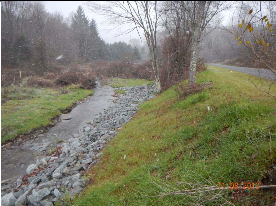
Photo 4: Looking downstream from right streambank after construction of rock rip rap along the streambank.
