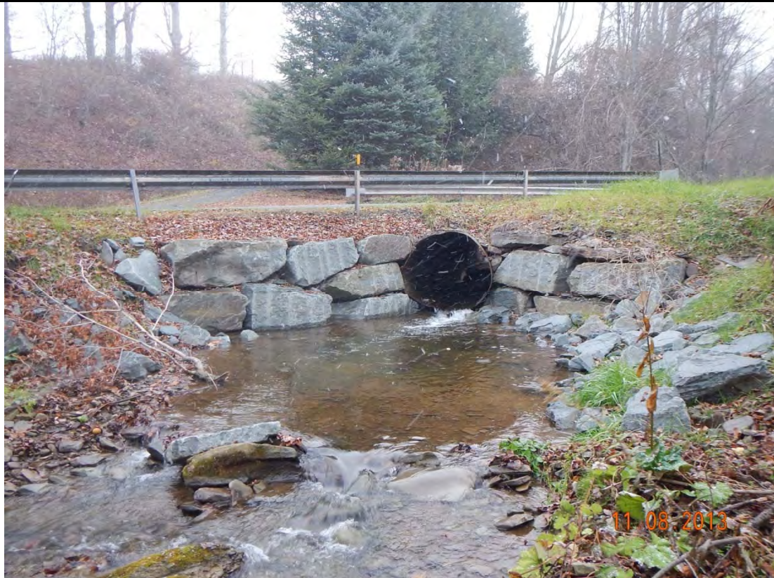
Photo 8: Looking upstream from MacGibbon Hollow culvert after construction of stacked rock headwalls.
