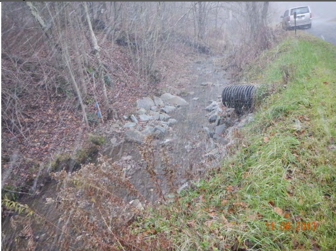
Photo 12: Looking downstream from right streambank after construction of culvert outfall protection and hardened riffle structure.
