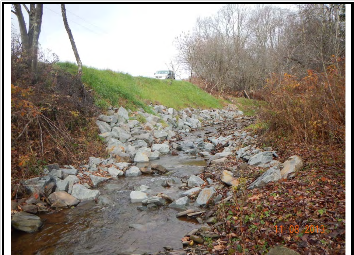
Photo 15: Looking upstream from left streambank after construction of rock rip rap and hardened riffle structure.
