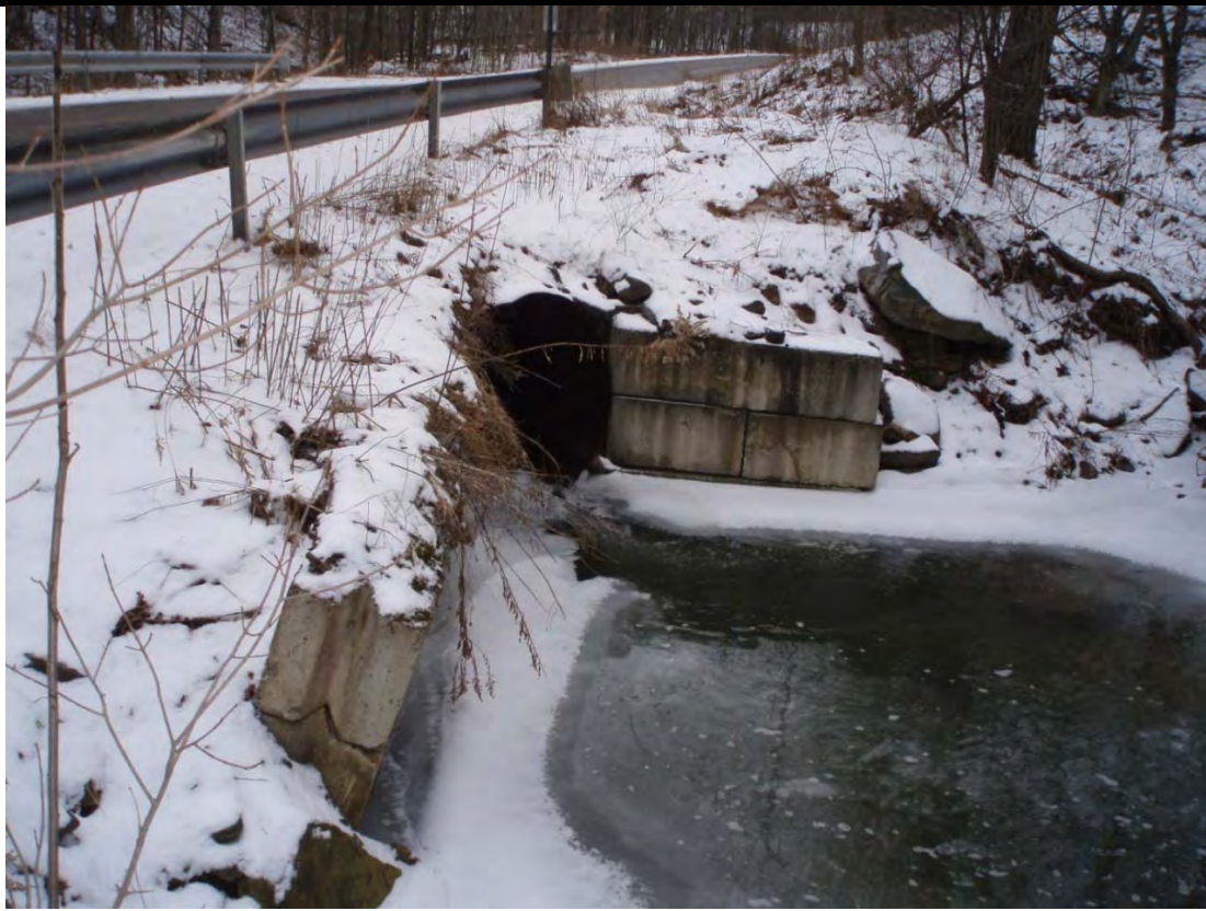
Photo 5: Looking at culvert along MacGibbon Hollow Road with headwalls that are failing.
