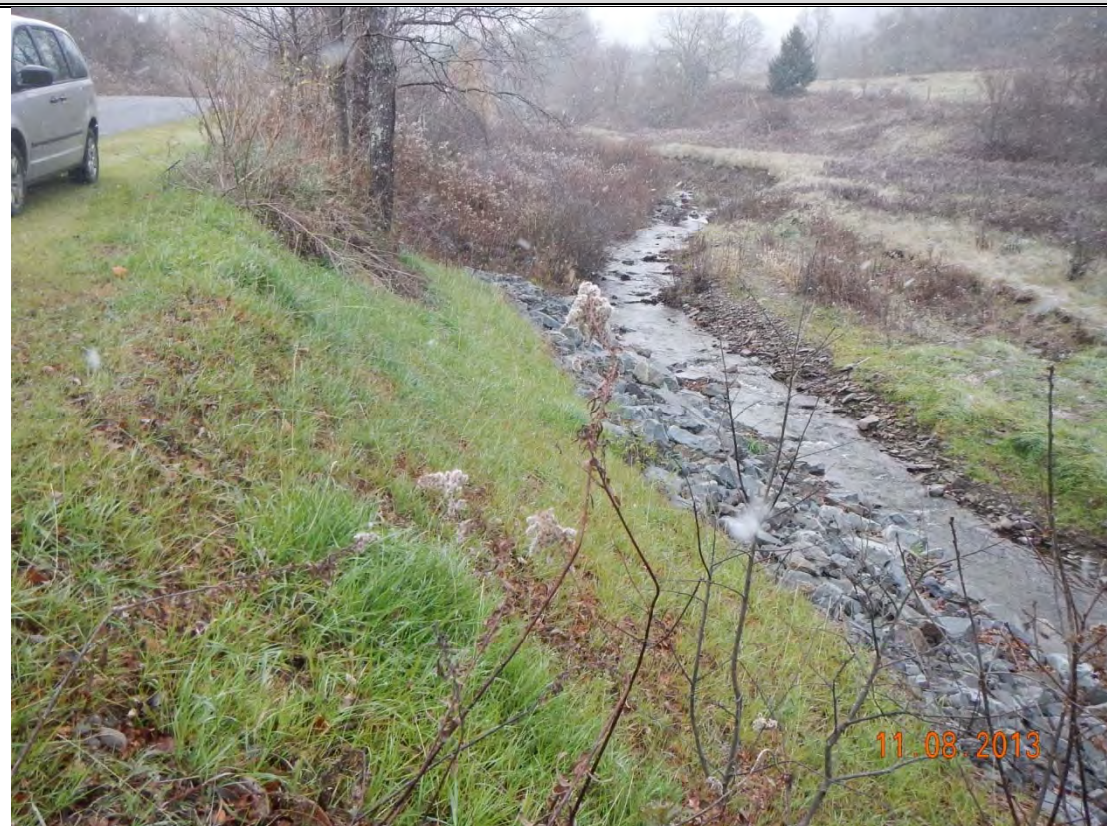
Photo 2: Looking upstream from MacGibbon Hollow Road after construction of rip rap along the streambank and floodplain on the left streambank.
