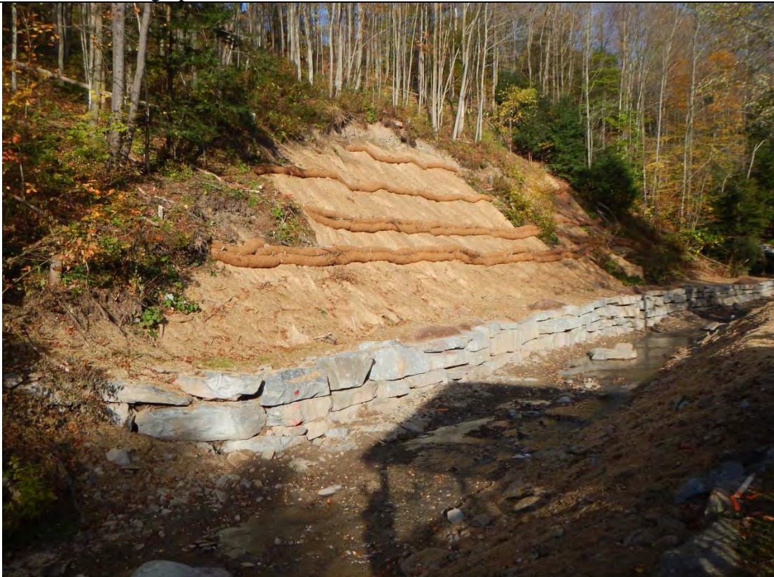
Photo 4: Looking upstream at the lower section of Site #3 after construction of rock wall, hardened riffle and erosion control.
