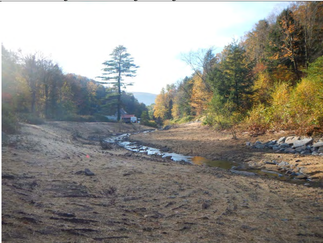
Photo 10: Looking downstream at Site #6 after construction of rock weir structures and stream channel relocation..
