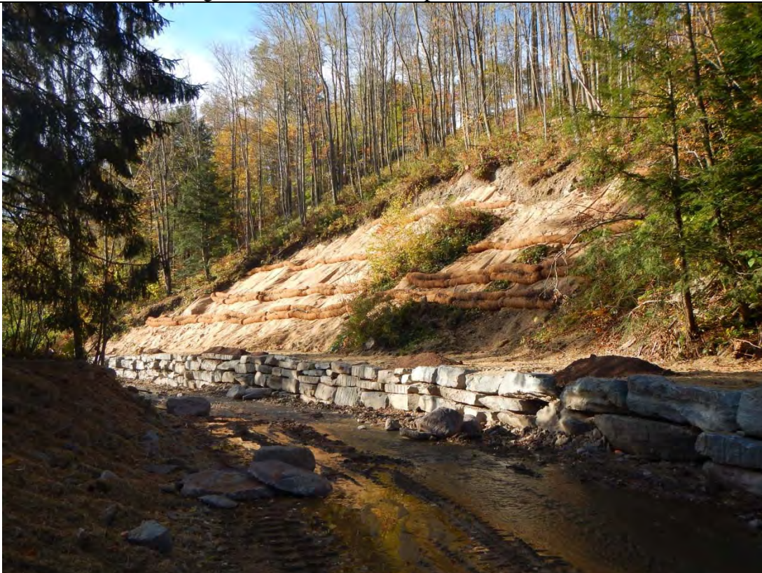
Photo 2: Looking downstream at the lower section of Site #3 after construction of rock wall and erosion control.
