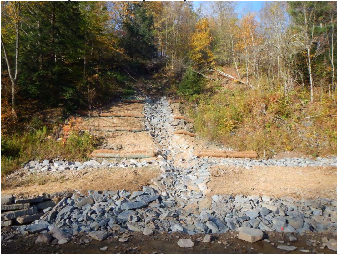
Photo 8: Looking downstream at Site #5 after construction of stacked rock wall, rip rap, drainage ditch and erosion control.
