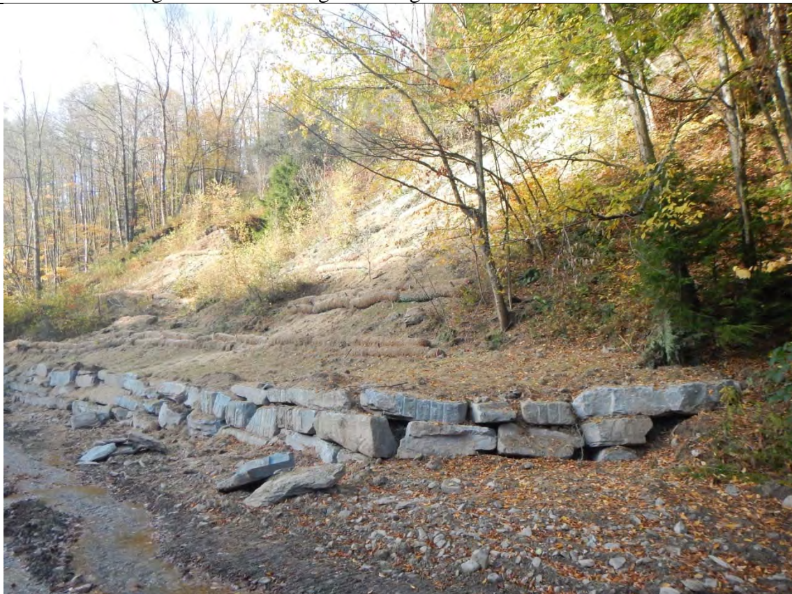
Photo 6: Looking downstream at Site #4 after construction of stacked rock wall and erosion control.
